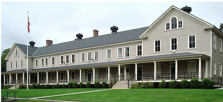
Figure 1: Modern view (facing northwest) of the Artillery Barracks at Fort Vancouver National Historic Site. This is a large U-shaped building, and the south-face of the building is currently shown. The location of the NCO Staff Quarters and privy, the focus of this study, is underneath the east wing (right side of the photo). Photo by author.
